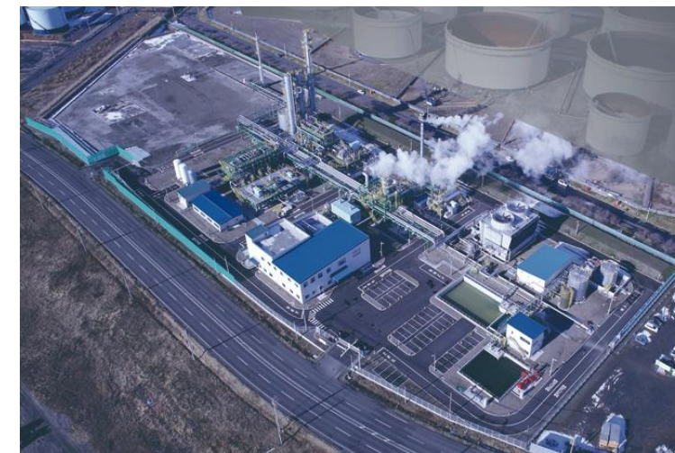
Tomakomai CCS Demonstration Facilities Source: JCCS
