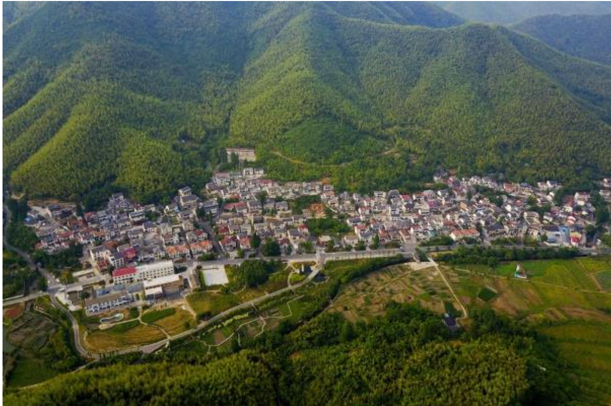
Figure 14 Yucun Village has committed itself to become a Carbon Neutral Village
