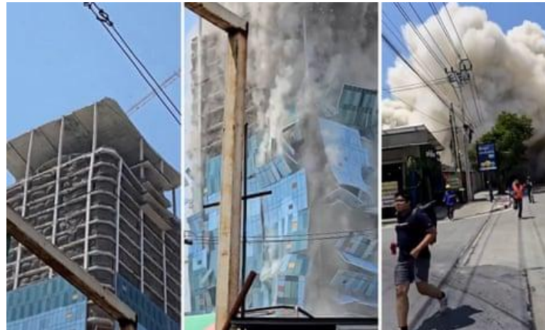
Figure 2: A tower block under construction in Bangkok collapsed from the earthquake 6 .
