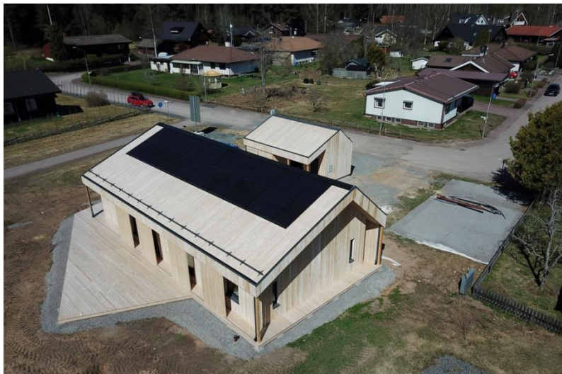
Figure 23 Villazero exterior with solar panels located in Borlänge, Sweden 105
