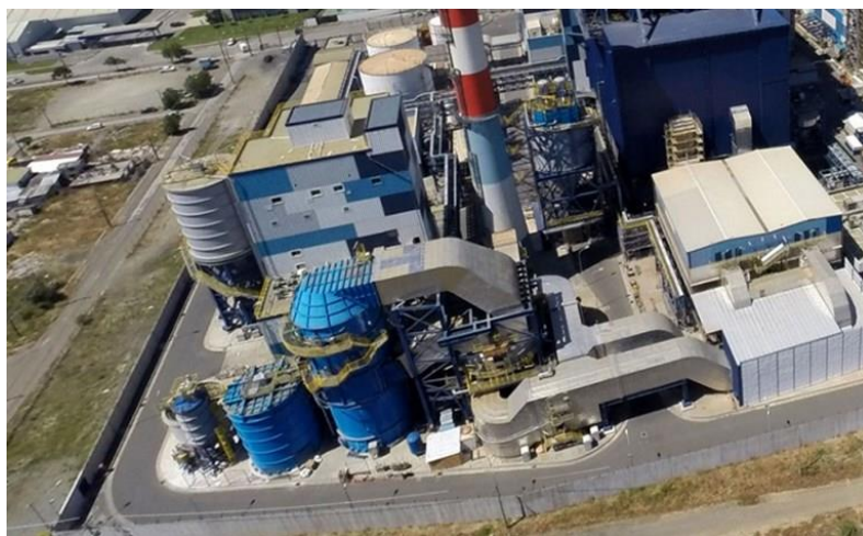
Figure 6 Enel Chile decommissioning plant
