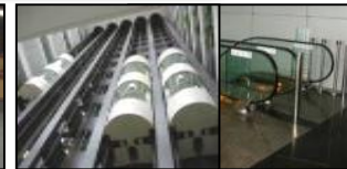
Lift/ Escalator Installation
